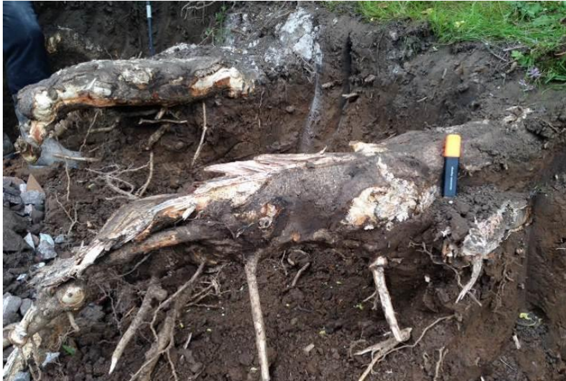
Plate 13. Structural roots severed just below the surface during excavations
