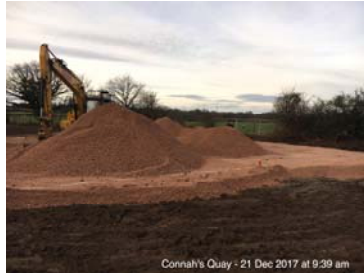
Stoning up ground to level
