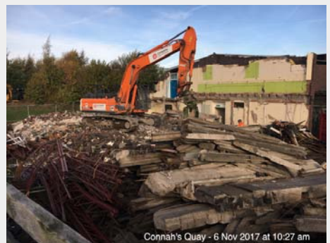
Machine demolition of old Design Technology block to the rear of the school
