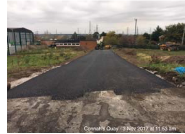
Temporary Access road
