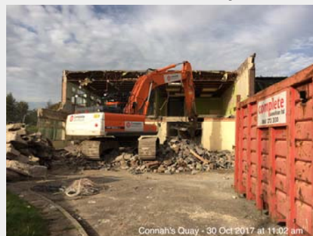
Machine demolition of old Design Technology block to the rear of the school
