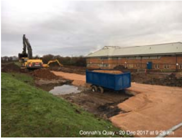
Reduced level dig and stoning up
