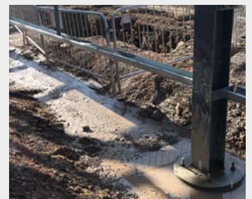
Grouting of steel bases
