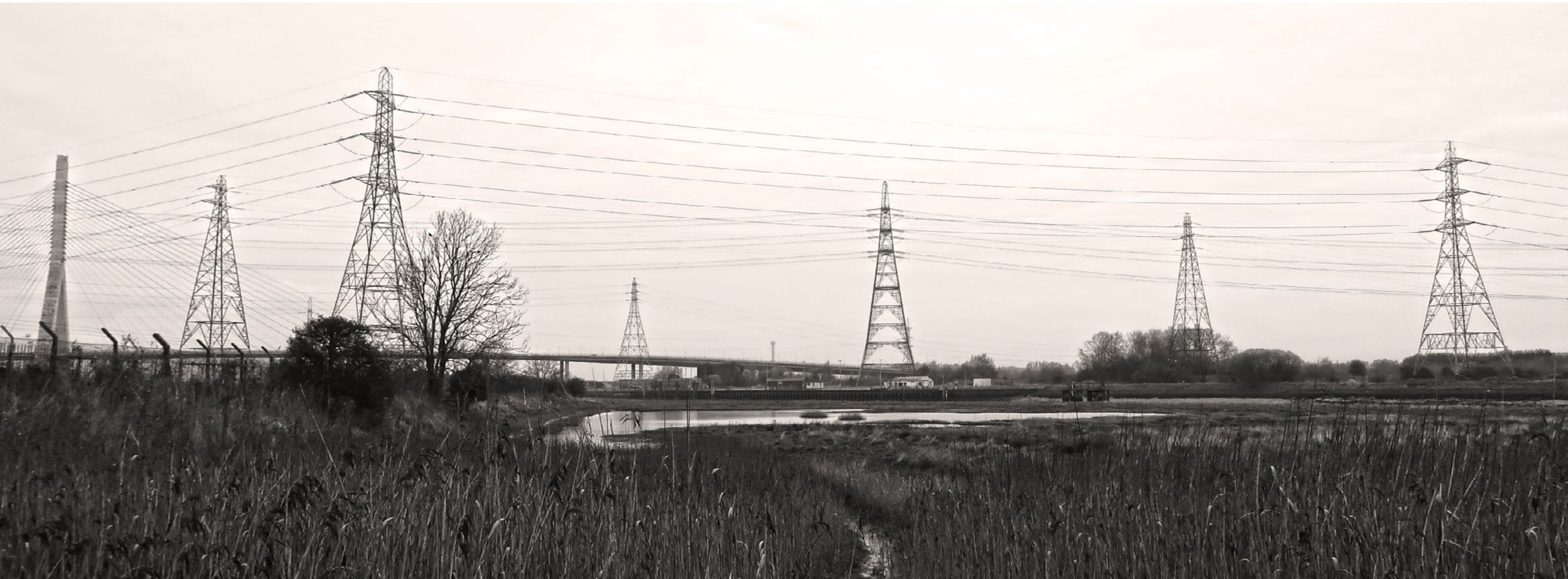
Fig 5.01: View of the site
