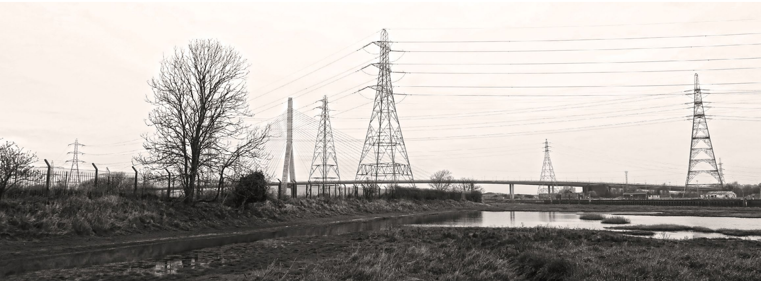
Fig 1.01: View of the site
