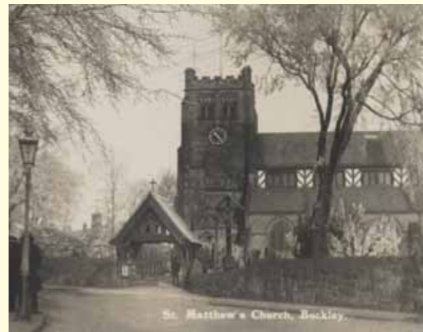
Saint Matthew's Church - c.1920 / Eglwys Sant Matthew - c.1920
