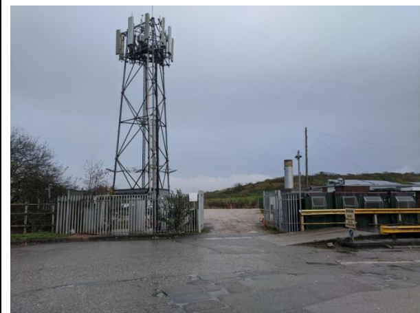
Photograph 2: view of rear of Site hardstanding area.
