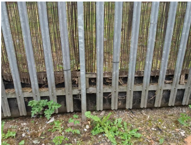
Photograph 6: Existing amphibian exclusion fence in place at base of perimeter fence of Site
