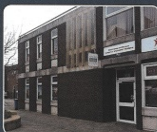
Mold Library Earl Road Mold CH7 1AP
