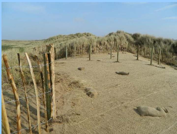
The picture shows an example of working with natural processes by raising the level and reinforcing the natural coastal sand dune system which will ultimately protect the village of Talacre.
