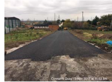
Temporary Access road
