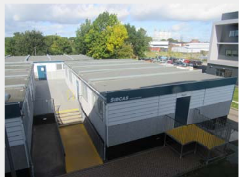
Temporary classroom set up
