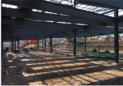
Ground floor slab preparation
