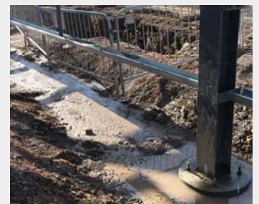
Grouting of steel bases
