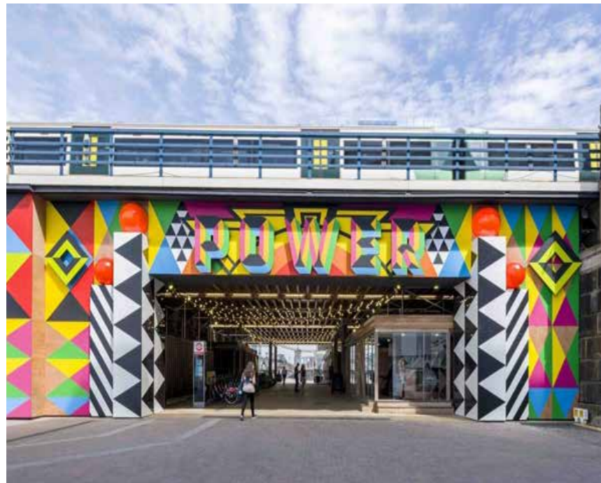
Opportunity to use art to enhance railway bridge
