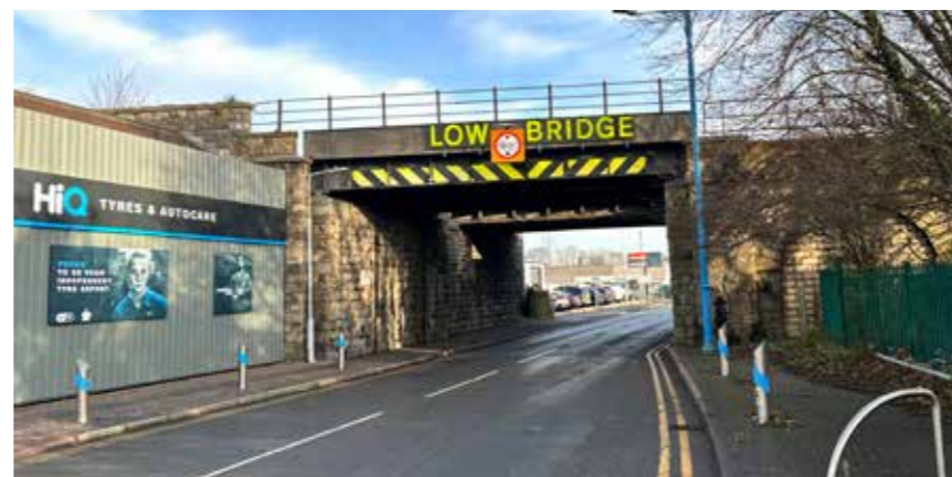
Existing eastern gateway
