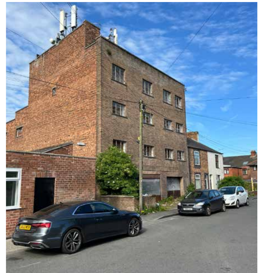
.....and derelict buildings
