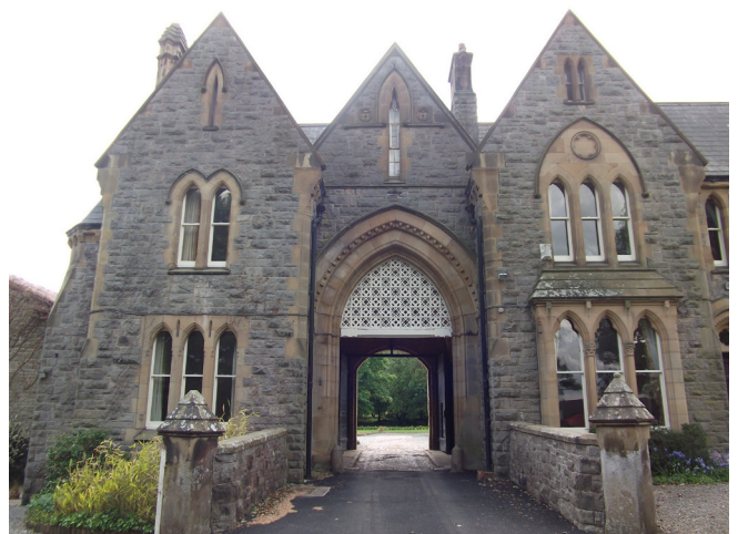
» Former Prison Gatehouse & Residence, Mold
