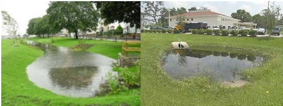
Figure 3.10 Drainage led SuDS Detention and Retention basins 32
