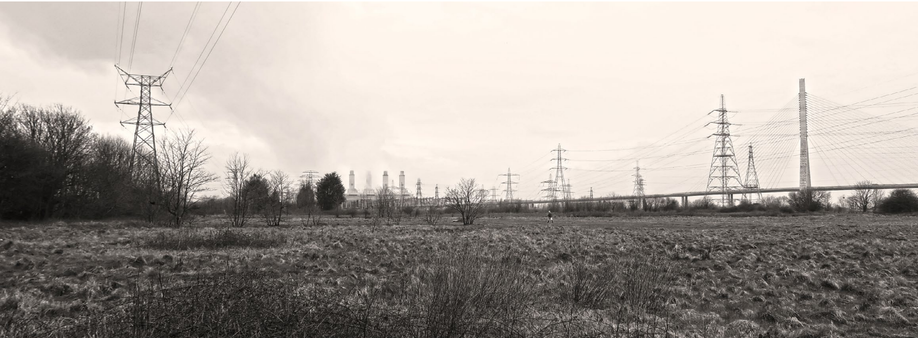
Fig 6.02: View of the site
