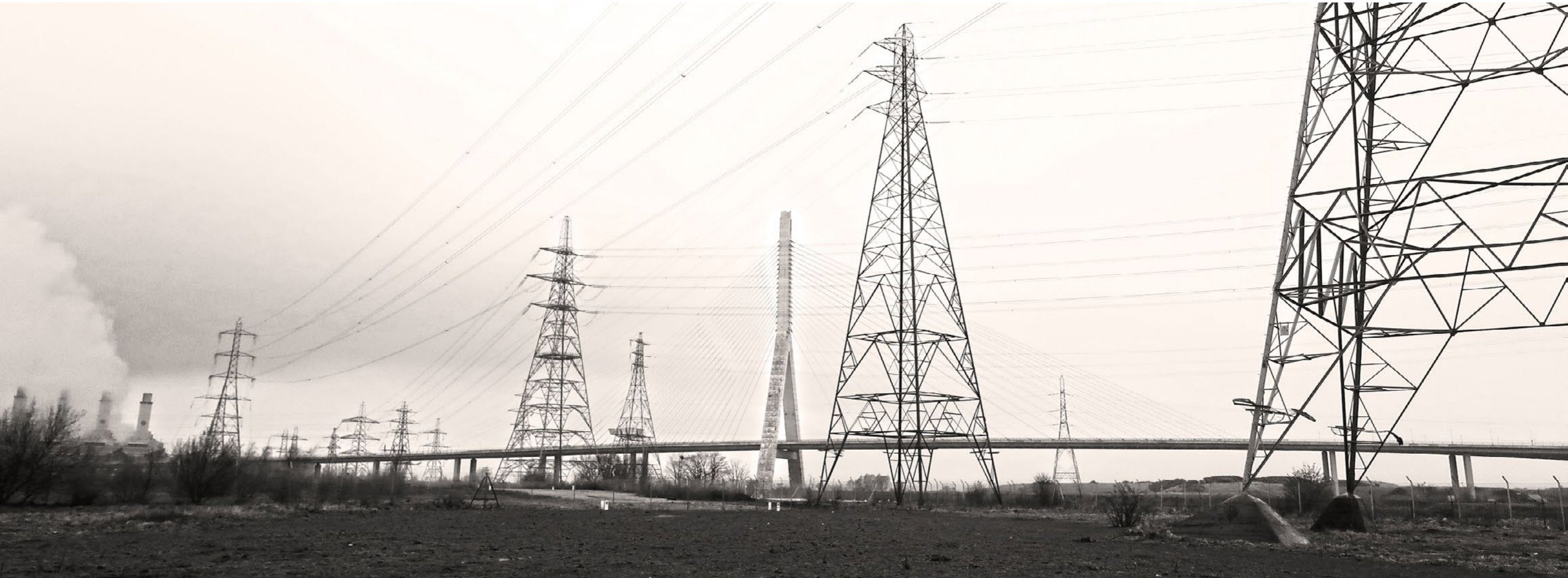
Fig 2.02: View of the site
