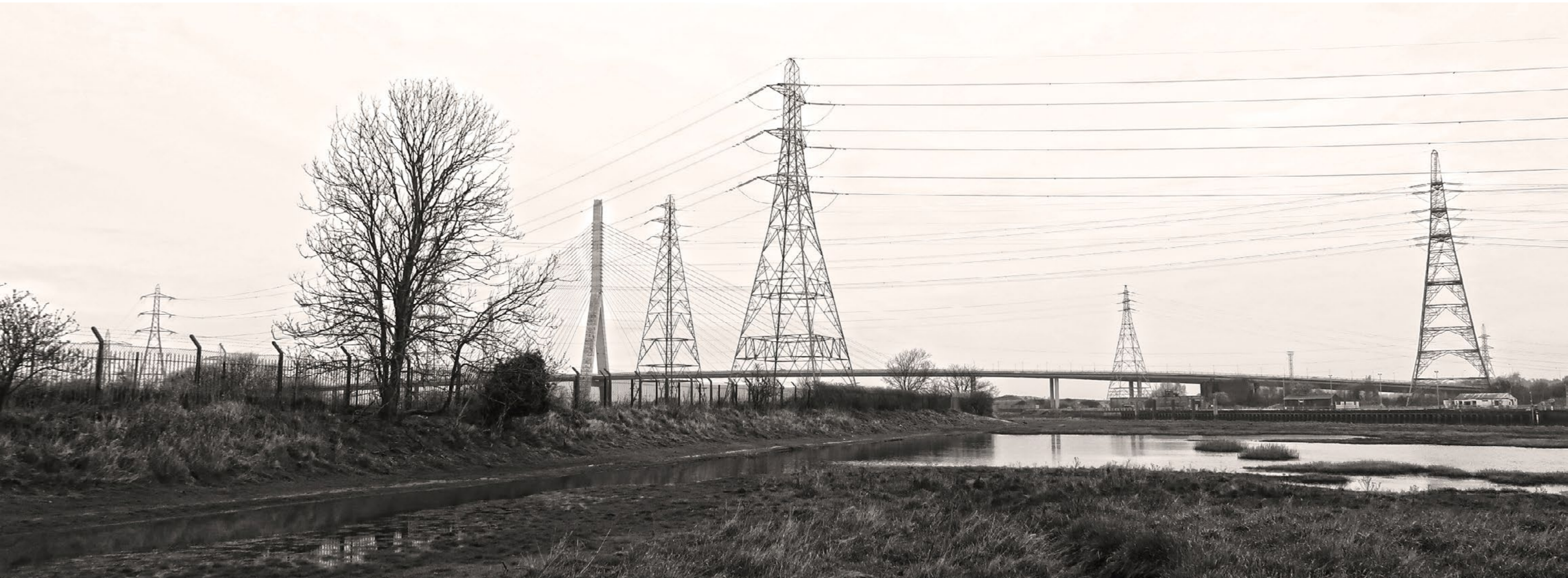
Fig 1.01: View of the site
