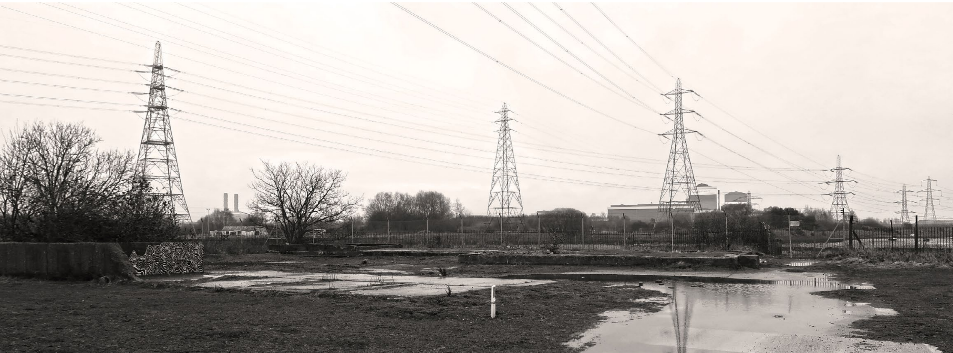
Fig 6.01: View of the site
