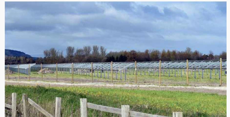
Figure 4. Typical view of solar farm during installation
