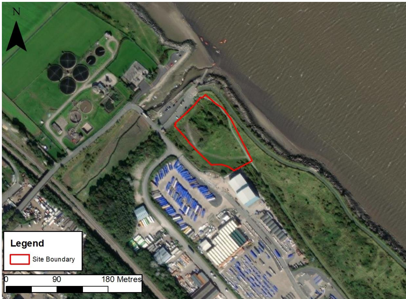
Figure 4-1 Aerial imagery of the site
