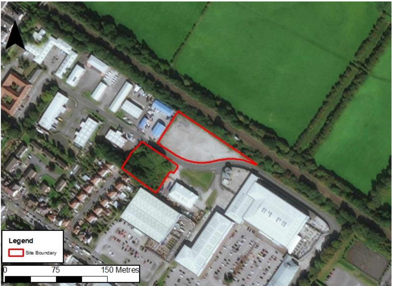
Figure 9-1 Aerial imagery of the site
