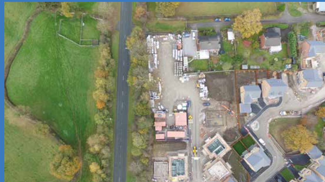
View of A550 bypass and Groves development
