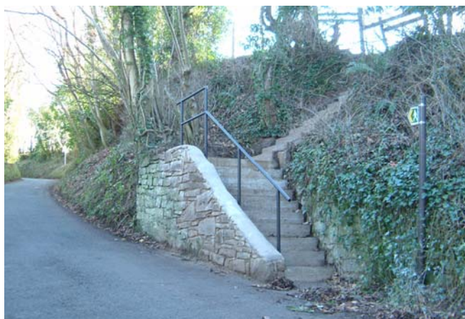
Public Footpath No. 6D Mostyn (formerly Whitford) (NGR 3160 3789)
